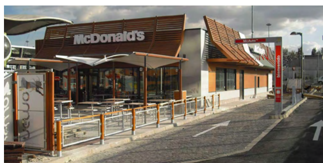
Construction of the first "folded" McDonald's restaurant on Avenida de los Poblados, Madrid.
