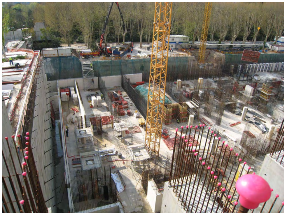
The museum's structure.
